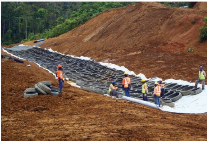
Construction of a drain using Ecoflex units at the Komo Airfield
