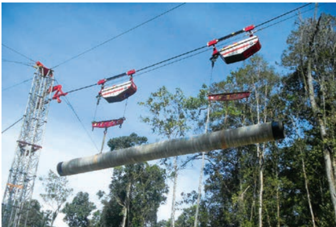
A pipeline segment being transported using the teleferic cable
