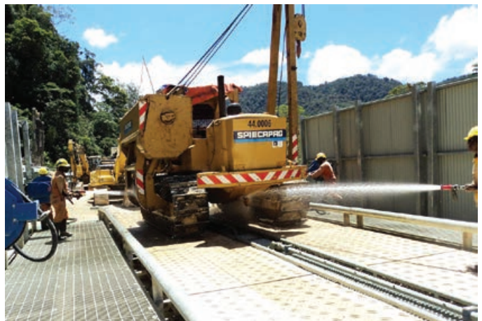
Equipment being washed at the Hides Permanent Vehicle Washdown Facility
