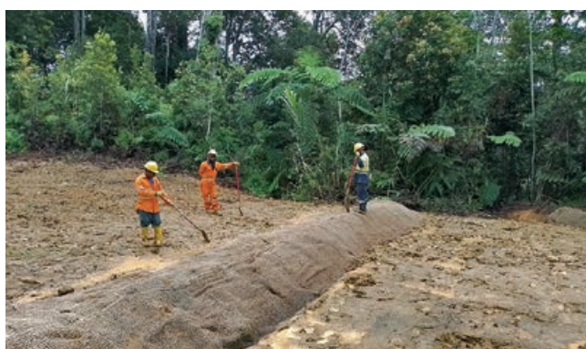
Reinstatement works at Kilometre Point 100
