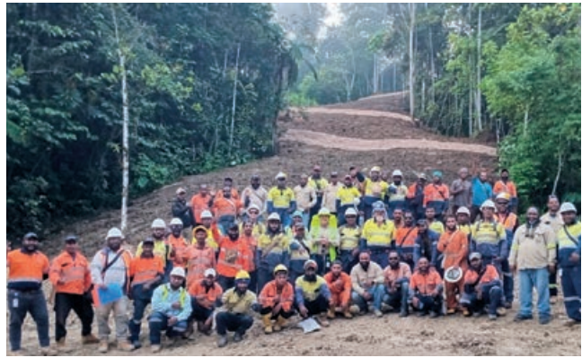
Celebrating successful completion of all earthquake recovery works along the pipeline ROW at Kilometre Point 100
