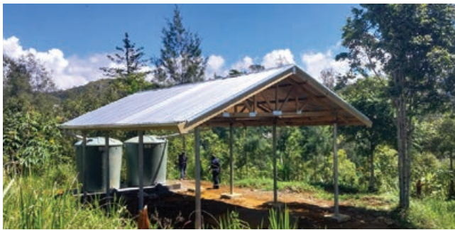
Water catchment structure constructed at Kulu Village
