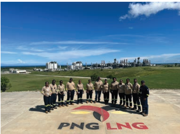
EMPNG’s above field workforce on a site tour at the LNG Plant
