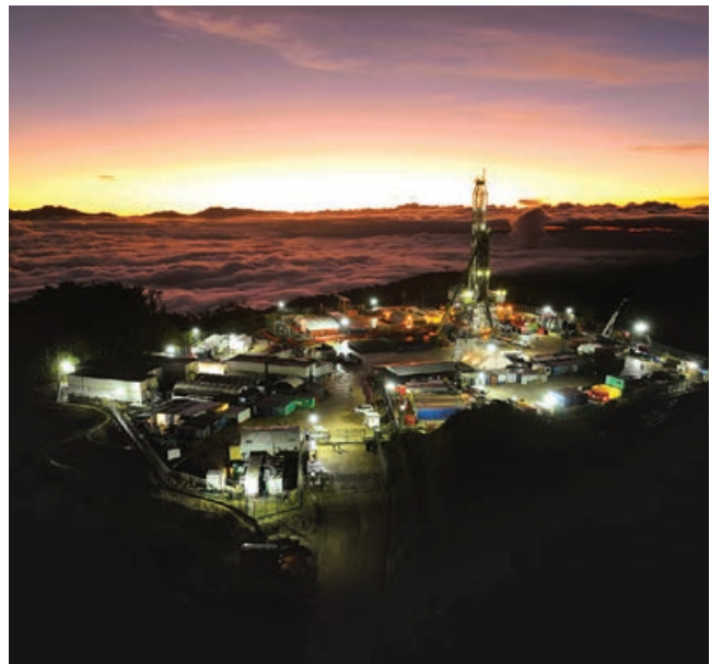
Nabors International’s Rig 702 at Hides Wellpad F during the Hides F2 well drilling campaign
