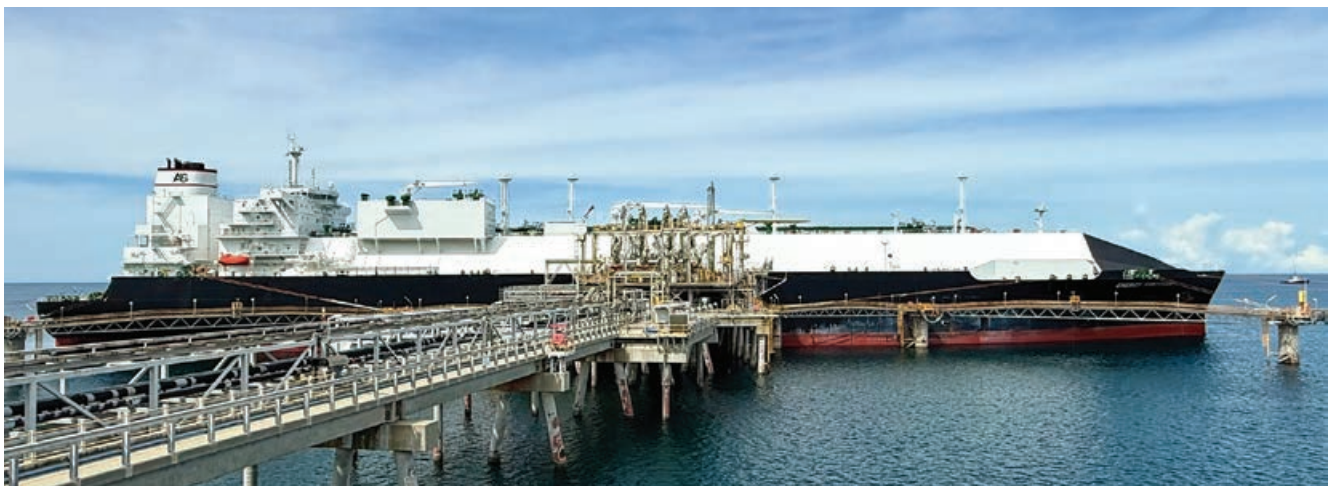
LNG vessel, Energy Fortitude berthed at the LNG Plant Marine Terminal jetty to receive the 116 th cargo for 2025
