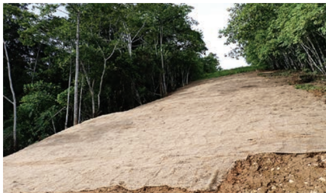
Jute mesh installation at Kilometre Point 98 on the pipeline ROW
