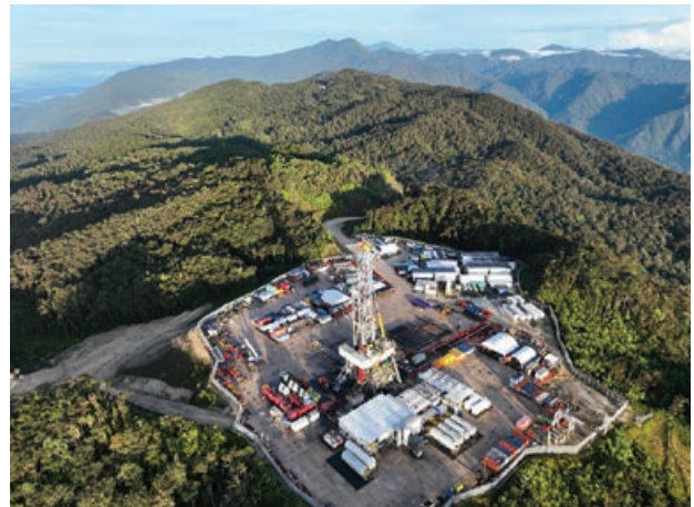
Aerial view of Hides Wellpad F
