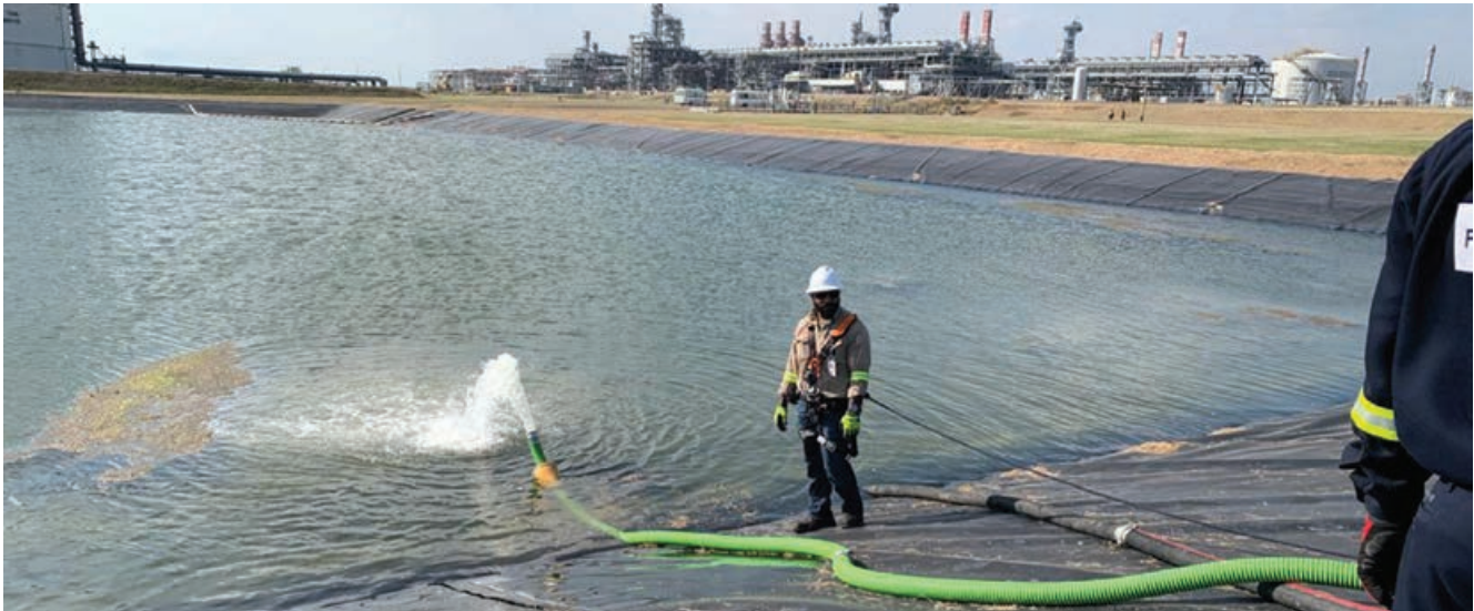
EMPNG Safety and OIMS Supervisor, Isaac Maima, conducts aeration at the LNG Plant retention pond
