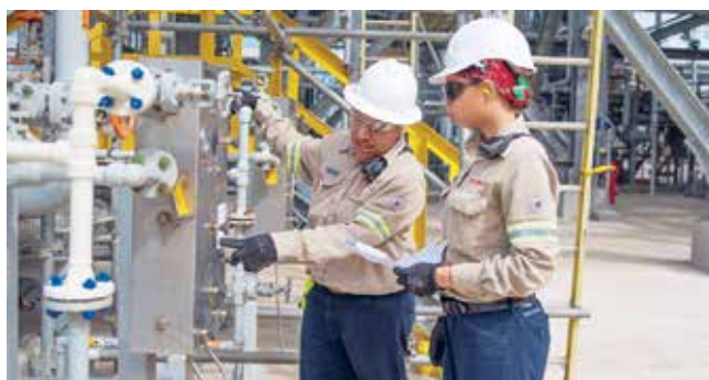
Plate 5.5 – Level 2 Operations Technician, Eunice Isaac, assisting Level 1 Operations Technician, Ramona Terence, with taking an amine sample
