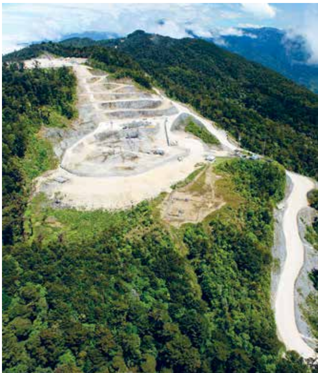
Plate 7.8 – Hides Wellpad Access Road leading to Hides Wellpads E and F
