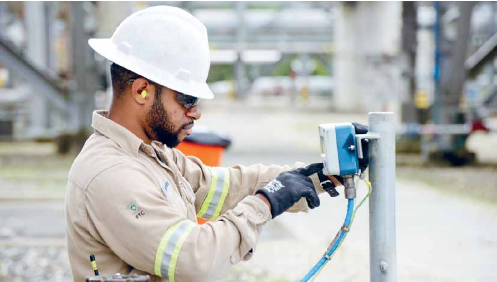
Plate 8.1 – EMPNG Electrical Technician, Yasi Koriem, working at the HGCP
